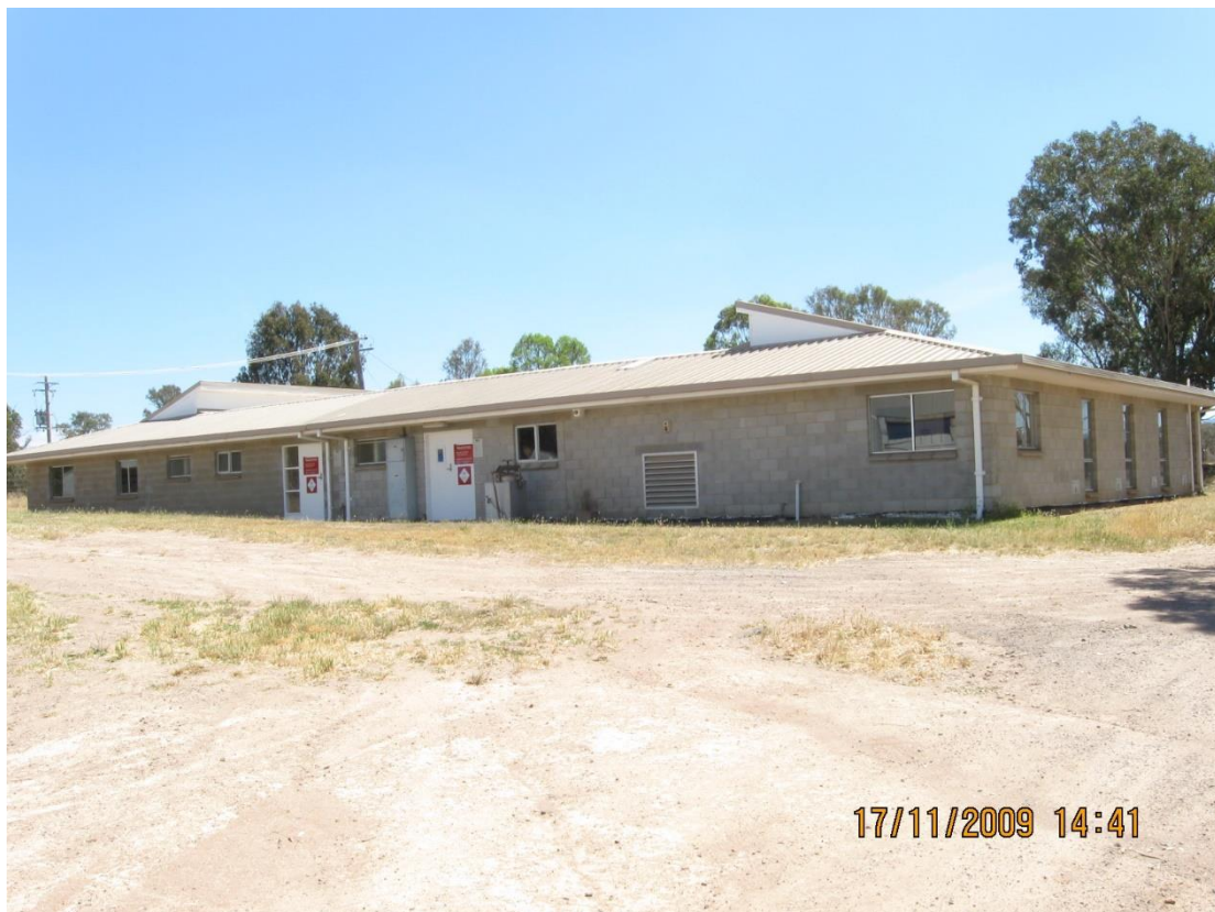
Photograph 01 - View of the Animal Breeding Facility Building SV07, emergency safe refuge.
