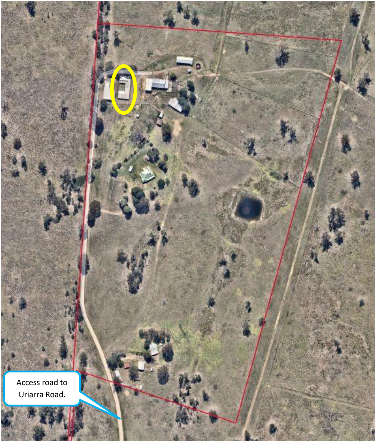
Image 06 – View of Lot 404 farm buildings and refuge building SV07.
