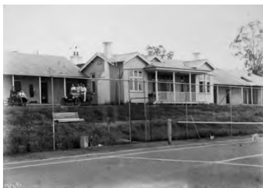
Heritage Childcare Centre at 15 Lennox Crossing (Building 75G)
