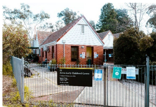
Acton Early Childhood Centre (Building 72)
