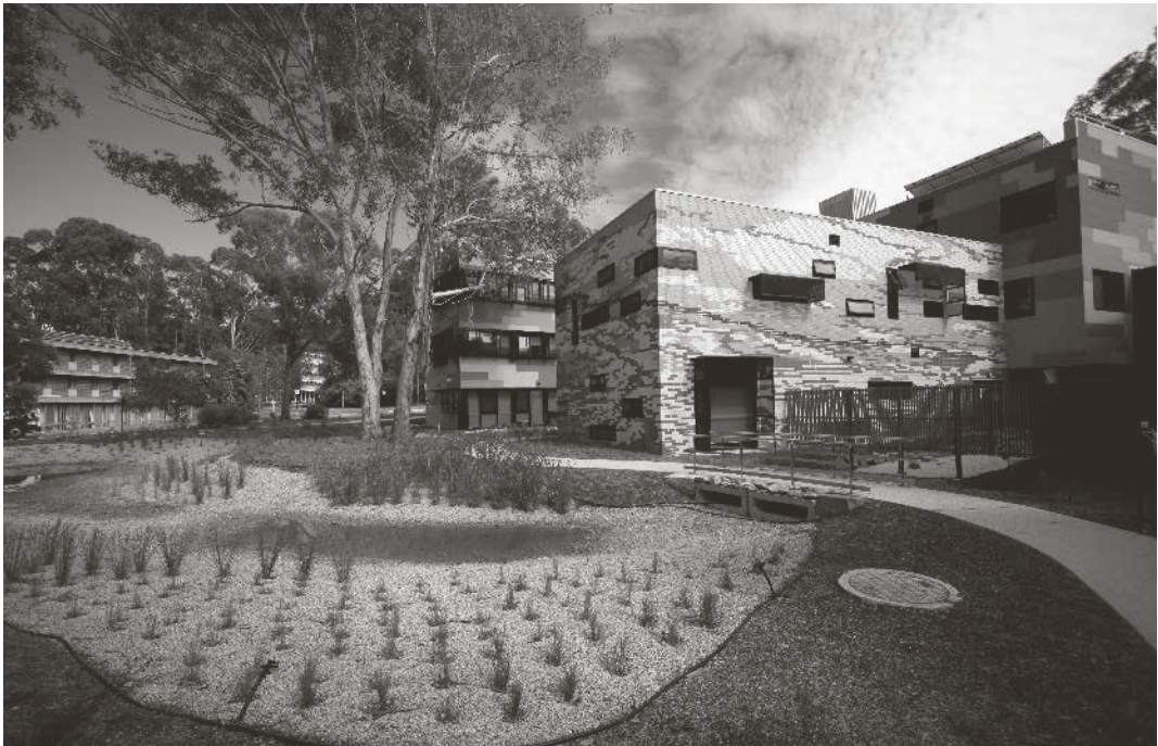
The new Frank Fenner Building features a range of sustainable design features, including a bio swale, which naturally filters run-off rainwater before it enters the nearby Sullivans Creek.
